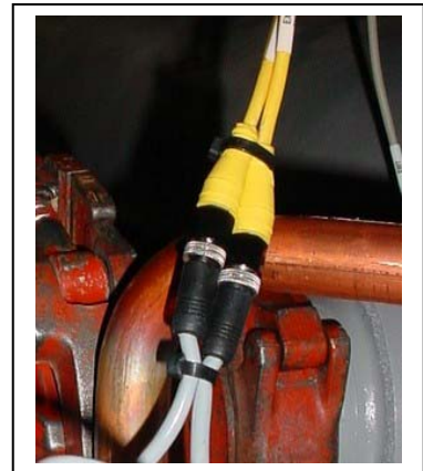
New EXV Cable Connector from 30RB660012
